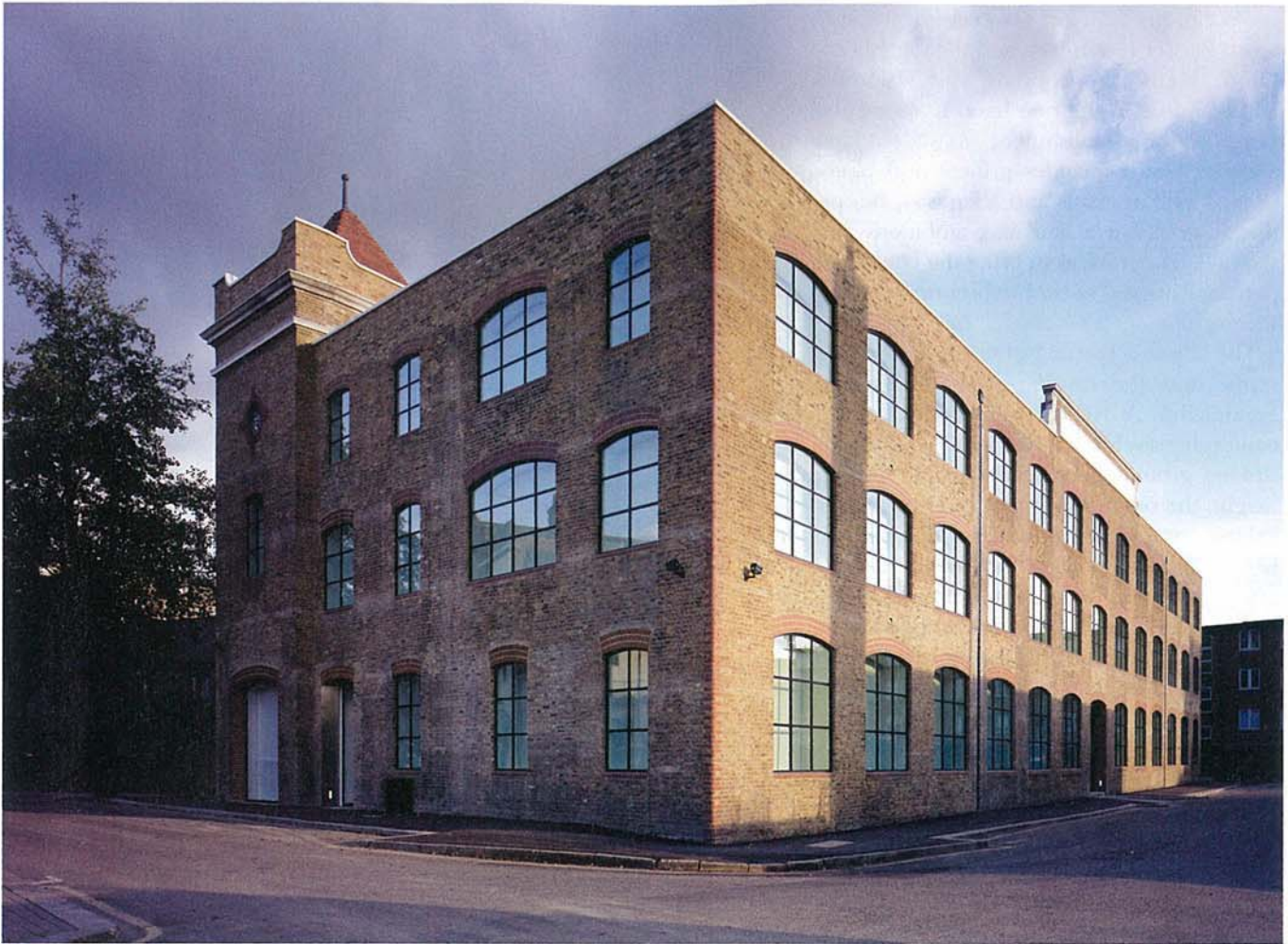
Above The renovation of the building included subtle but important adjustments to the facades. The height and spacing of windows was regularised, and large areas of masonry rebuilt. A proposal to use single sheets of glass in the windows was rejected by planners (ph: HB). Right The building before renovation. Built as a coachworks, it had more recently been used as offices by design and advertising agencies (ph: RD). Below North-south section, showing the trusses from which the upper floors are suspended. The two trusses also form the sides of two rooflights to the second floor.
