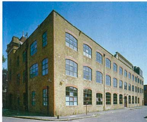
Above The renovation of the building included subtle but important adjustments to the facades. The height and spacing of windows was regularised, and large areas of masonry rebuilt. A proposal to use single sheets of glass in the windows was rejected by planners (ph: HB). Right The building before renovation. Built as a coachworks, it had more recently been used as offices by design and advertising agencies (ph: RD). Below North-south section, showing the trusses from which the upper floors are suspended. The two trusses also form the sides of two rooflights to the second floor.
